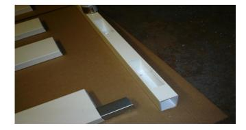
Add the glue to the other gate post the same way and insert the gate post onto the rails. Make sure it goes all the way in.
