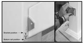
(3b) Place bracket covers on bottom rail. (Bracket covers may require additional modifications i.e. extending cutouts for pickets, and/or splitting covers along the score line.)
